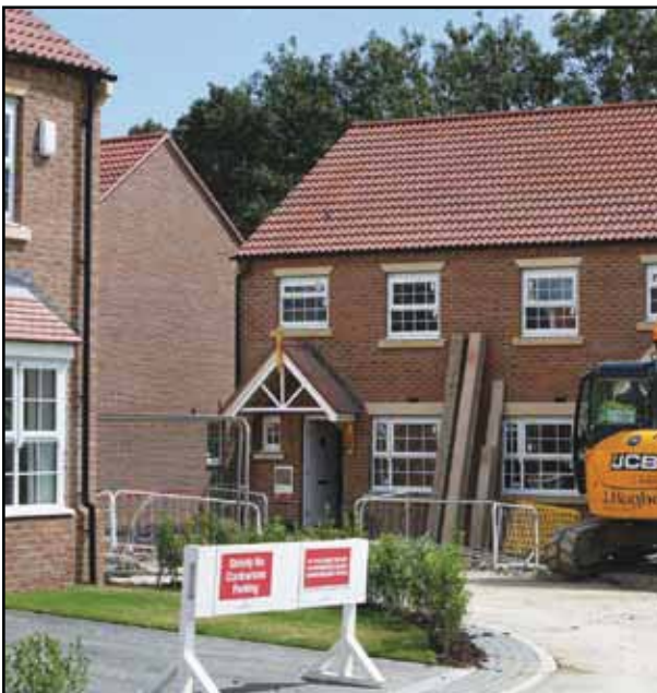
The Oaklands, building affordable homes in Easingwold
